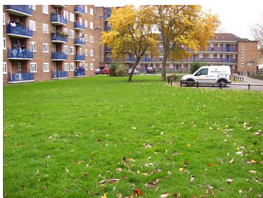
Frampton Park Estate, Hackney. Before
